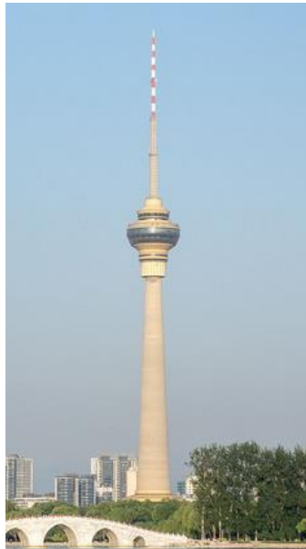
Central TV Tower, Beijing
